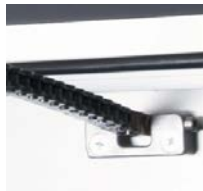
chain operator attached to frame
