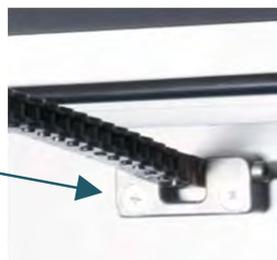
chain operator attached to frame
