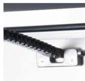
chain operator attached to frame
